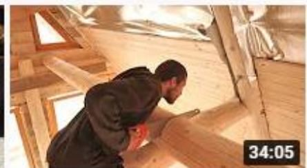
Off Grid LOG CABIN Build / Setting LOFT LOGS in Plac...
