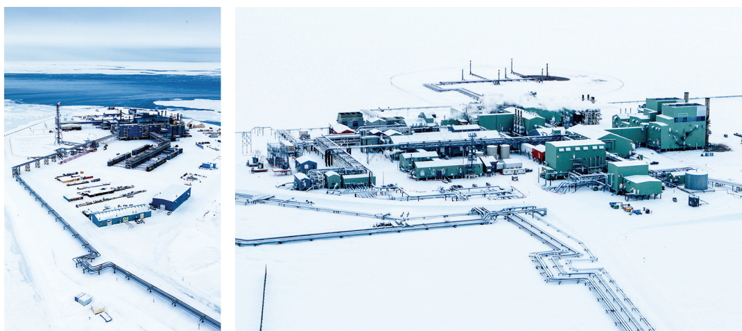
Figure 19 : British Petroleum, Endicott Offshore Field et BP Alaska's Prudhoe Bay operations 85
